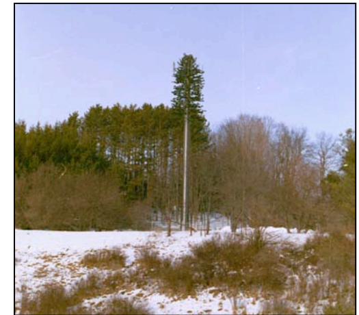
Photos (top to bottom): The Marcy-South power line has had a negative visual impact on the community - this Plan opposes situating like facilities in the Town; cellular communication tower in the hamlet of Livingston Manor, NY that is disguised as a pine tree. The cell tower design works since there are pine trees on this site. Cell towers have also been situated on silos.
