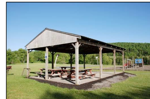
Above (top to bottom): New Lisbon Community Park that is located behind Town Hall in the Hamlet of Garrattsville. The park includes a baseball diamond, picnic pavilion and tot lot for community residents.
