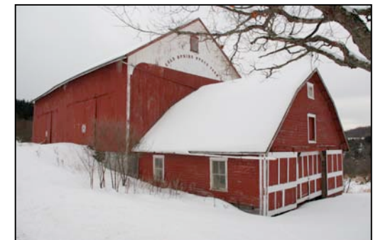
Above (top to bottom): Historic barn on CR 12 in the hamlet of New Lisbon; barn on Jones Road on property surrounded by Texas Schoolhouse State Forest; and barn at Cold Spring Stock Farm on Texas Road. Each of these barns helps to define the rich agricultural history of the Town and efforts to preserve these structures are strongly supported by this Plan.
