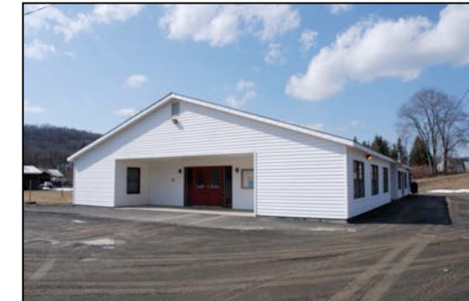
Above (top to bottom): Garrattsville Fire House that is home to the Garrattsville Fire Department and Ambulance Corps; County Highway Barn on Route 51; and New Lisbon Town Hall in the hamlet of Garrattsville.
