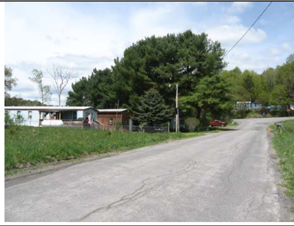
CR 15 looking north to CR 14 intersection
