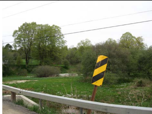
Coles Bridge Rd, millpond site on Butternut Creek
