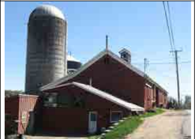
4241 NY 51, main barn on east side of highway
