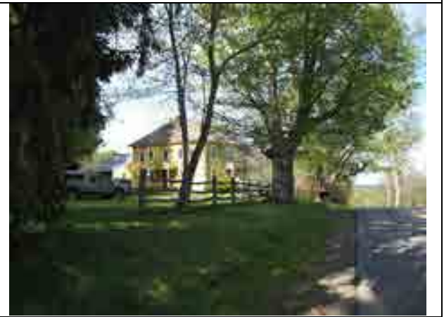
1115 CR 14, Greek Revival-era house
