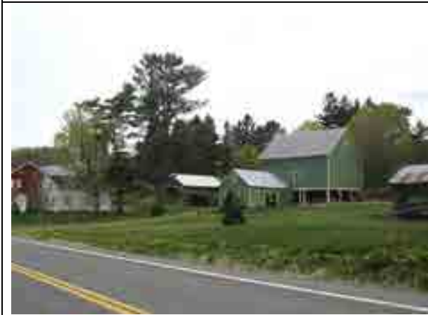
3927 NY 51, barns and outbuildings
