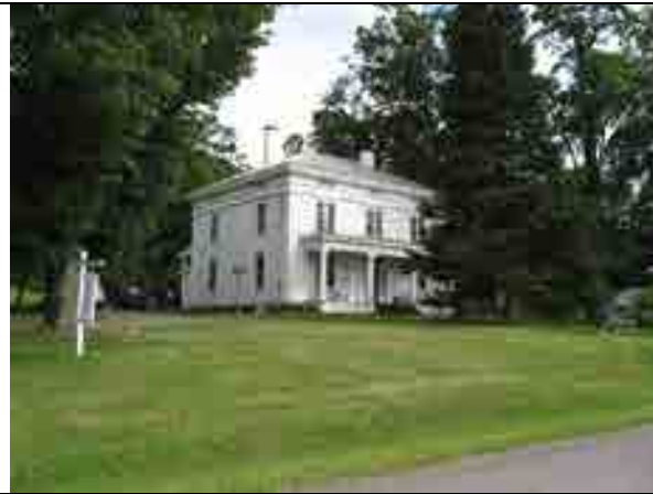
830 Pegg Rd (built ca.1835; individually NRE)
