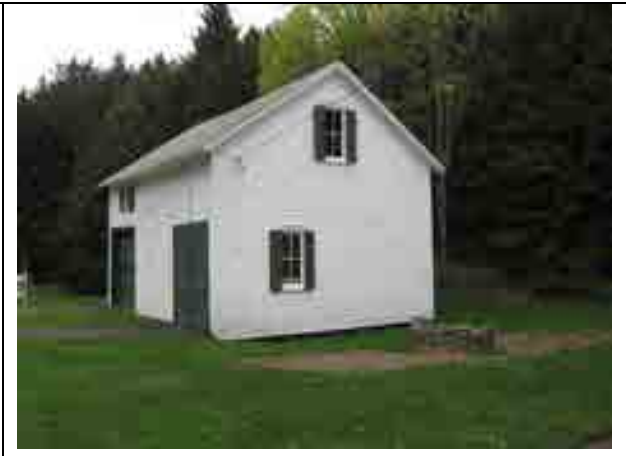
4411 NY 51, outbuilding (built ca.1880)
